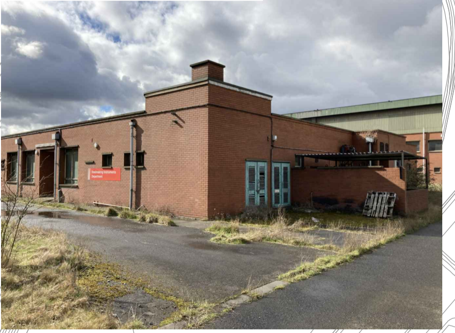
CONCAST CANTEEN AND OFFICES
